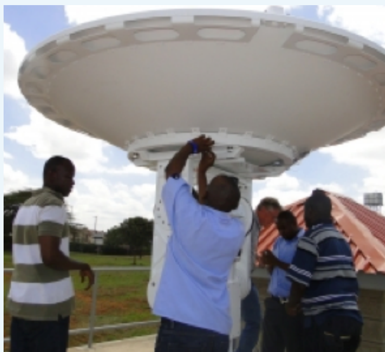
RCMRD's Data Officers James Mumina and Kenneth Kasera working on fitting and orienting the MODIS antenna/receiver in the confines of the Centre
