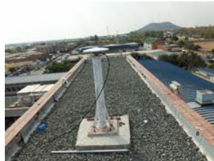
Figure 2: An installed Trimble NetR9 GNSS Receiver
